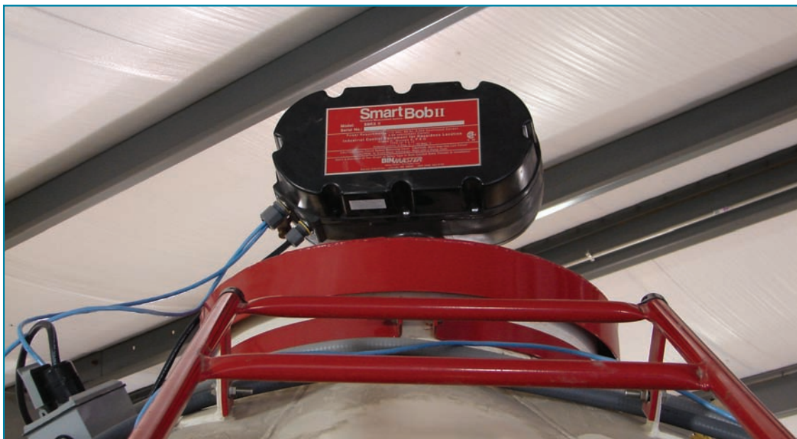
The SmartBob II is a cable-based system that is useful in corn or soybean applications where level measurements only need to be made a few times a day.
