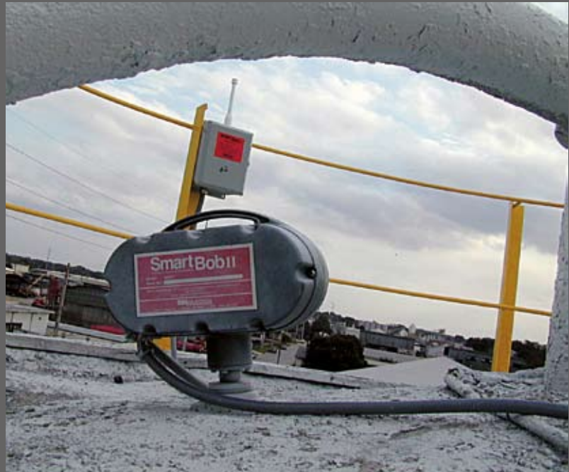
SmartBob is ideal for single point level measurement where silo levels need to be taken periodically throughout the day.
