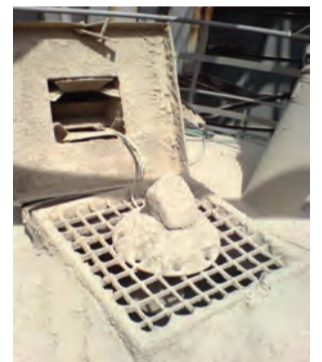
Although the 3DLevelScanner is coated in dust, the inside of the device is clean and operable.
