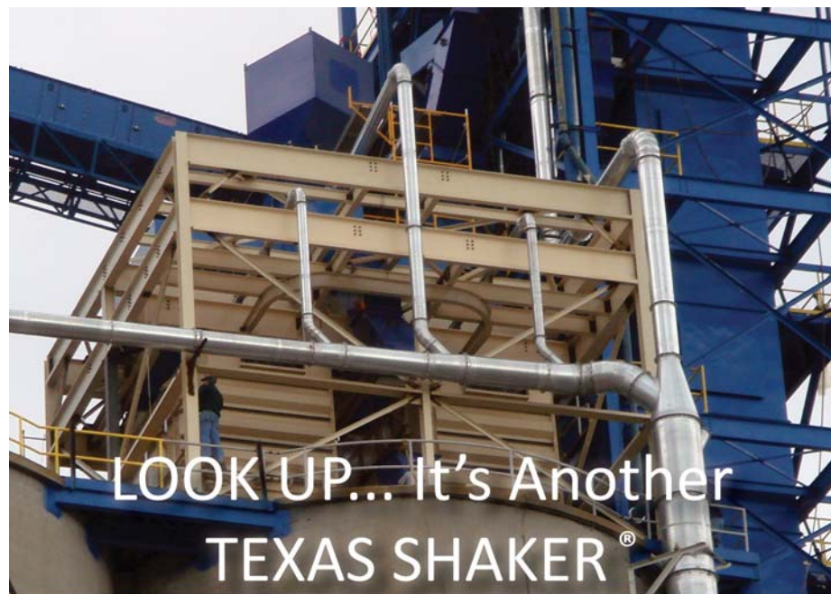
New 7,500-bph Zimmerman tower dryer sits adjacent to an older 3,500-bph model. The legs to the left were upgraded to 10,000 bph and a Union Iron Works tower with staircase was added.
