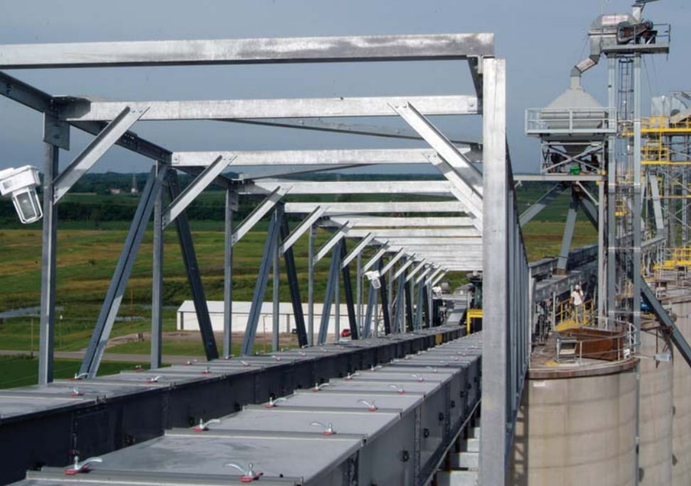
Twin Intersystems enclosed belt conveyors run out to the new storage from a pair of existing, upgraded Honeyville legs. However, the Intersystems gravity screener in the background is new.
