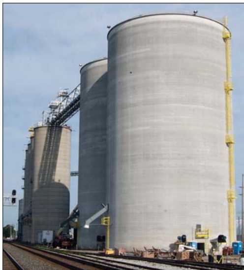
Closeup of two new 435,000-bushel slipform concrete tanks at the east end of the complex, built in 2009-10 by Adams Building Contractors.
