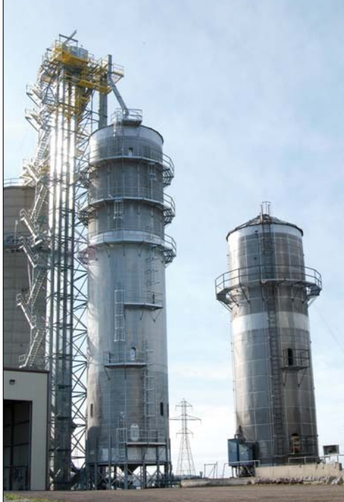
New 7,500-bph Zimmerman tower dryer sits adjacent to an older 3,500-bph model. The legs to the left were upgraded to 10,000 bph and a Union Iron Works tower with staircase was added.
