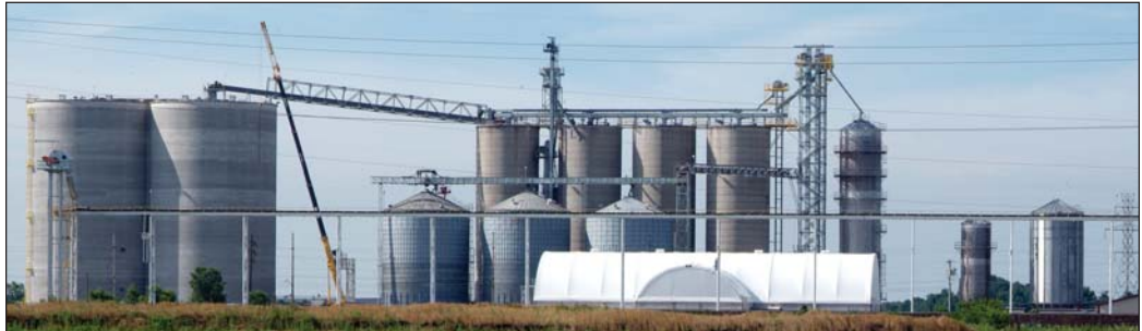
DeBruce Grain Inc.'s new rail-loading terminal on the Norfolk Southern in New Carlisle, IN, its first rail terminal east of the Mississippi. Photos by Ed Zdrojewski.
