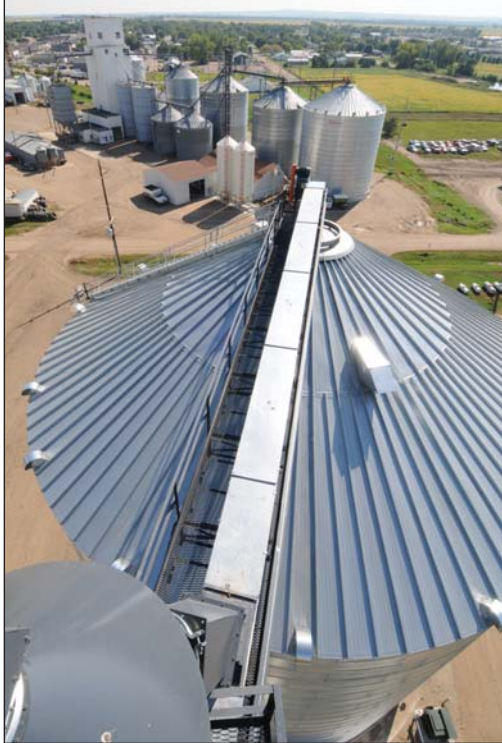
Overhead view of the 15,000-bph Schlager fill conveyor, with the rest of the Farmers Elevator facility in the background.
