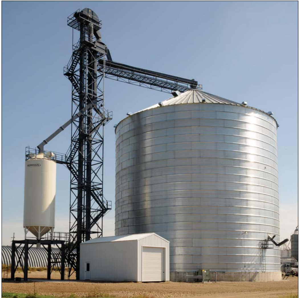
New 315,000-bushel steel annex at Farmers Elevator Co. of Platte, SD includes a Behlen storage tank, 15,000-bph Schlagel grain handling equipment, and 2,500-bushel Meridian surge tank. Photos by Bruce Selyem.
