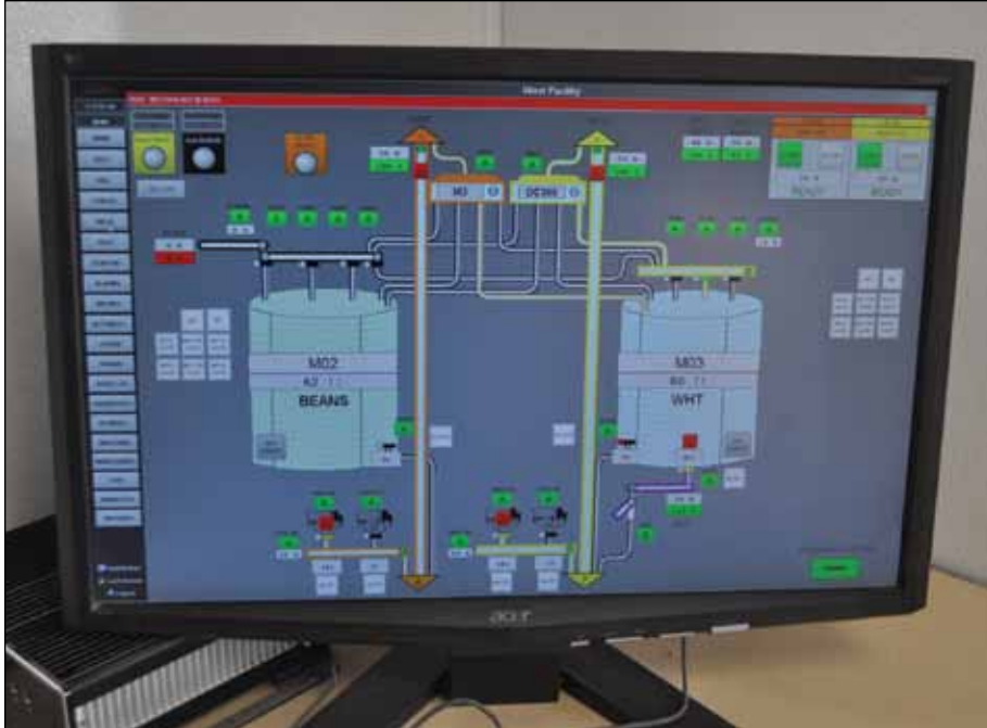
One of many screens available to elevator operators via a KASA control system shows the contents of two new jumpform concrete tanks and status of equipment serving those tanks. Additional photos by Ed Zdrojewski.
