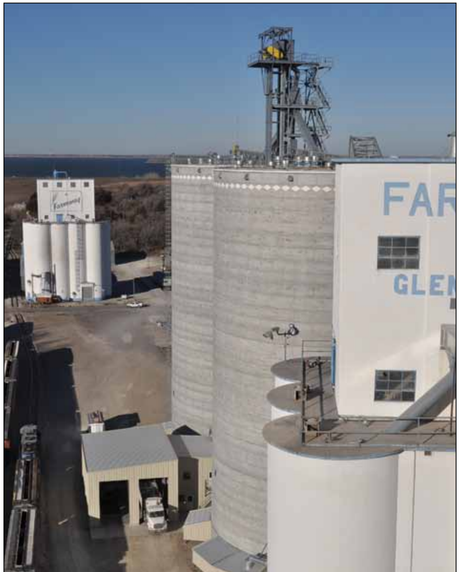
Another view of the expansion project at Glen Elder from the roof of the main concrete house, with new construction in the center of the photo.
