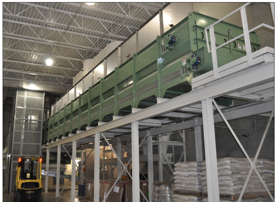
The mill's 63-foot-long CPM horizontal cooler is raised to provide additional storage space.
