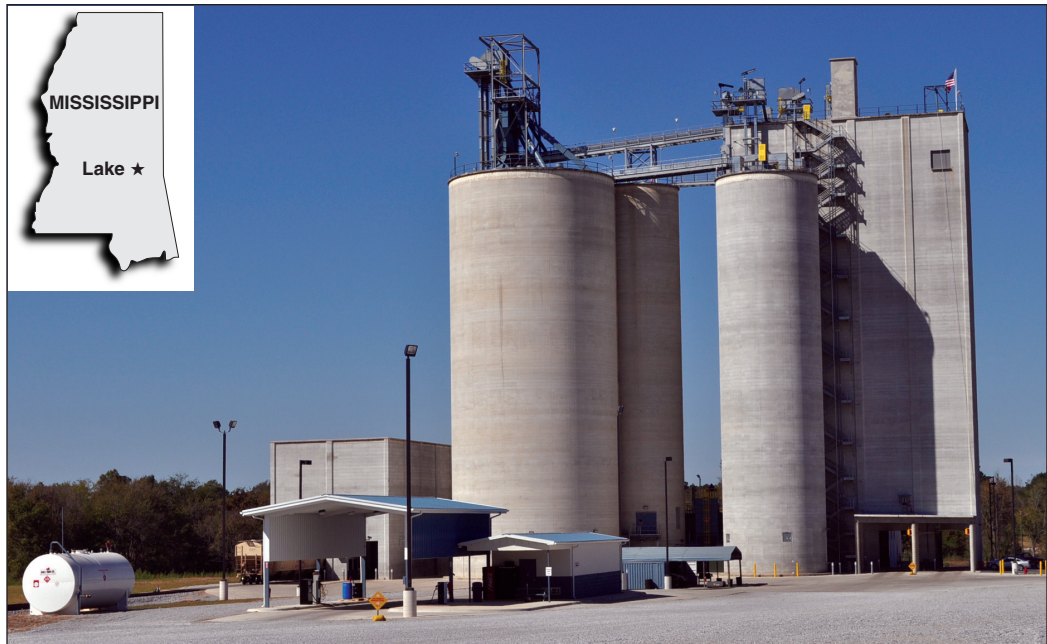
Peco Foods' new 8,800-tpw slipform concrete feed mill in Lake, MS designed to serve the Alabama-based company's poultry producers in Mississippi. Photos by Ed Zdrojewski.
