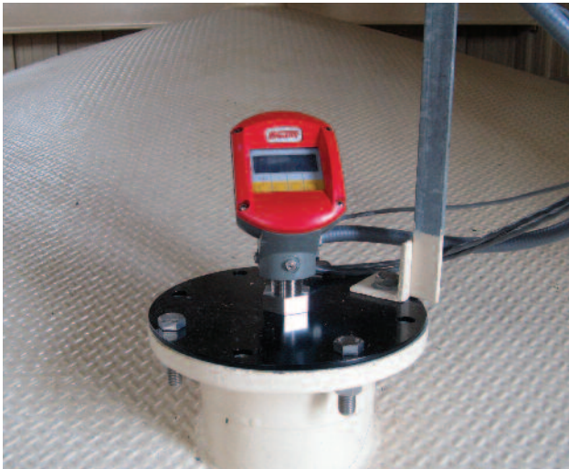
A 3D Scanner is a non-contact, dust penetrating devices that measures multiple points in the tank to provide greater accuracy.
