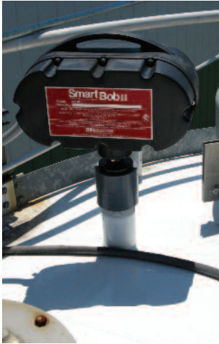
A bob-style sensor provides high accuracy when mounted near the outer perimeter of the tank.
