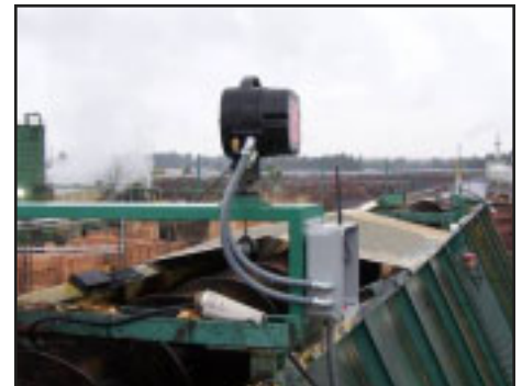
A SmartBob2 sensor installed on a chip bin at the Plum Creek sawmill in Columbia Falls, Montana
