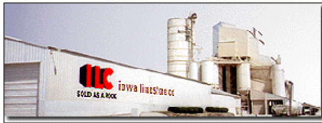
Iowa Limestone in Weeping Water, Nebraska
