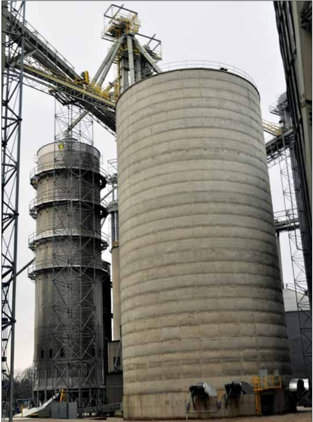
Installation at Sunrise Cooperative's Clyde, OH terminal includes a 250,000-bushel Hoffmann jumpform concrete silo, 10,000-bph Zimmerman tower dryer, and 15,000-bph Hawthorne-Seving wet and dry legs with six-hole Hayes & Stolz rotary distributor visible behind the tank. Photos by Ed Zdrojewski.
