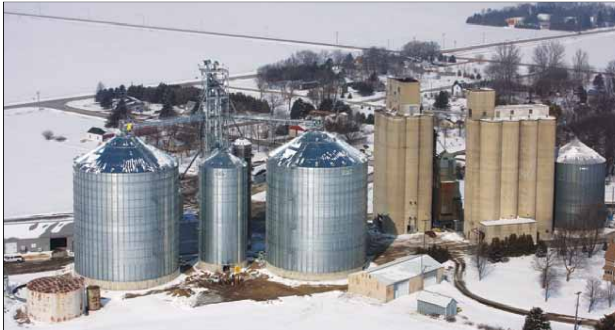
Five Star Coop's Burchinal location added two new 550,000-bushel steel tanks, a 110,000-bushel wet bin, 4,700 bph grain dryer, and a receiving pit in 2012. Aerial photo by JH Photography, Spencer, IA.
