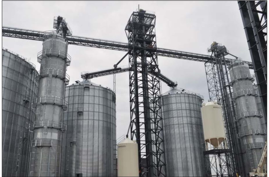
Key pieces of grain handling equipment include two Brock 4,700-bph dryers at right and left and three 20,000-bph Howell receiving legs at center, with Warrior towers and catwalks.
