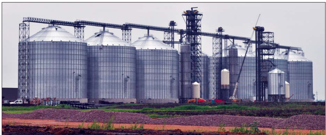
View of the Graceville terminal from the northeast showing all of the 5 million bushels worth of upright steel storage. Ground level photos by Ed Zdrojewski.
