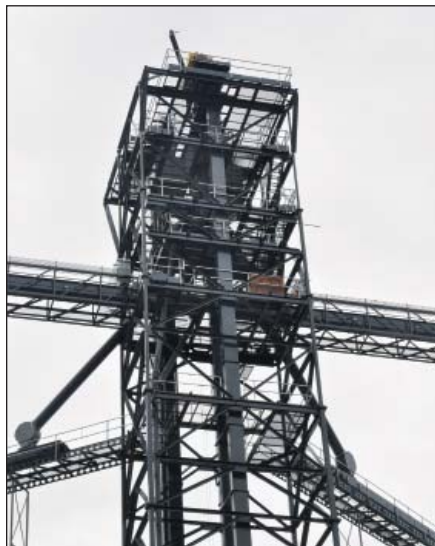
Receiving legs feed into a five-hole Schlegel electronic triple distributor.
