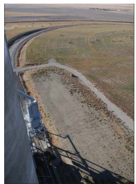
Overhead view of a 50,000-bph Intersystems bulk weigh loadout scale and an 11,500-foot, 120-railcar loop track running off a Burlington Northern Santa Fe main line.
