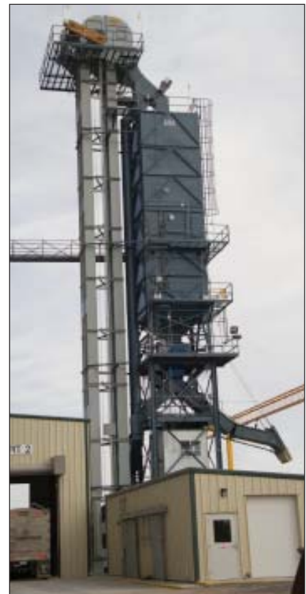
A C&A Scales bulk weigh scale with an extended upper gantry for rail loadout. Photo by Alex Lord.
