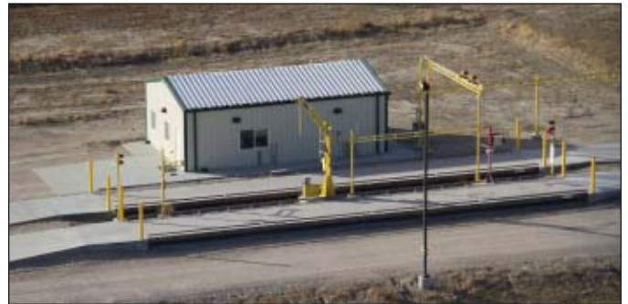
A separate scalehouse is equipped with two C&A scales and Gamet probe. Photo by Alex Lord.
