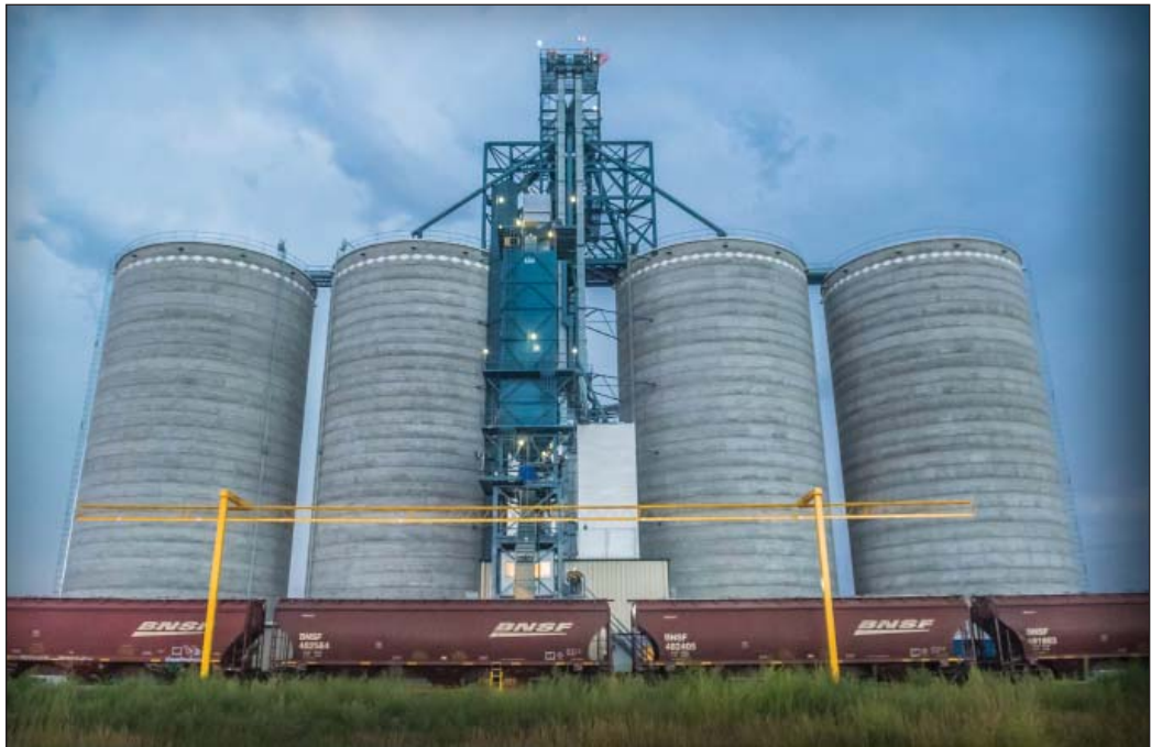
Frenchman Valley's new rail terminal in Culbertson, NE includes four McPherson Concrete silos holding 280,000 bushels each. Photo provided by Frisbie Construction Co. Inc.
