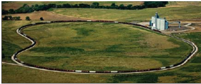
The shuttle terminal at Culbertson includes an 8,800-foot loop track. Photo provided by Frisbie Construction Co. Inc.
