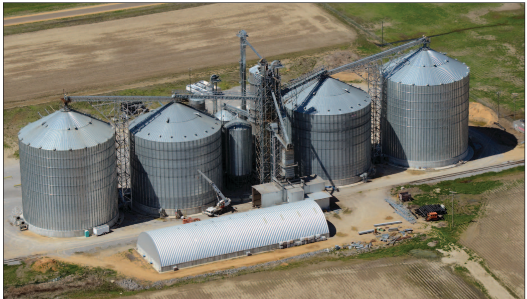
Express Grain Terminal LLC's 3.1-million-bushel rail terminal elevator at Sidon, MS features two new 775,000-bushel Chief Titan tanks at either end of the complex. Aerial photo by Greg Campbell, Madison, MS.
