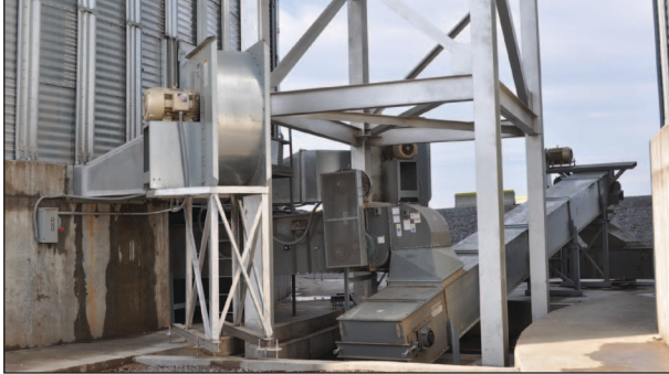
A set of 40,000-bph Hi Roller enclosed belt conveyors empty out the new tanks. Also visible is one of four 40-hp Caldwell centrifugal fans per tank. Ground-level photos by Ed Zdrojewski.
