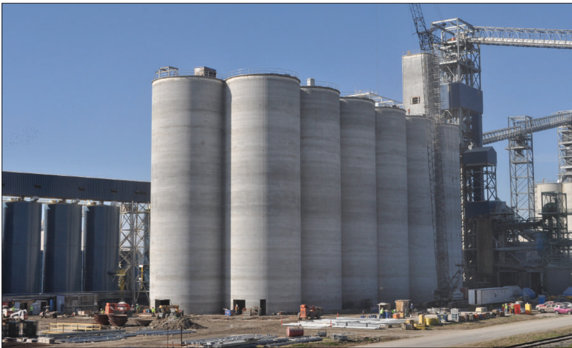
New 1.8-million-bushel slipform concrete annex under construction by Younglove Construction LLC in February 2014. Photo by Ed Zdrojewski.
