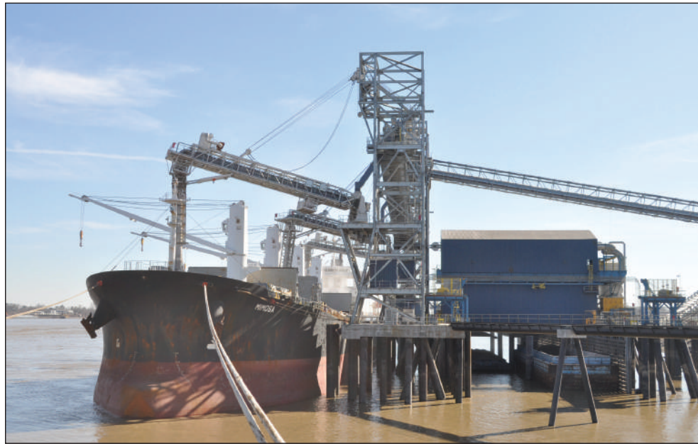
New berth on the Mississippi includes facilities for loading oceangoing vessels at the left and loading barges at right. Photo by Ed Zdrojewski.
