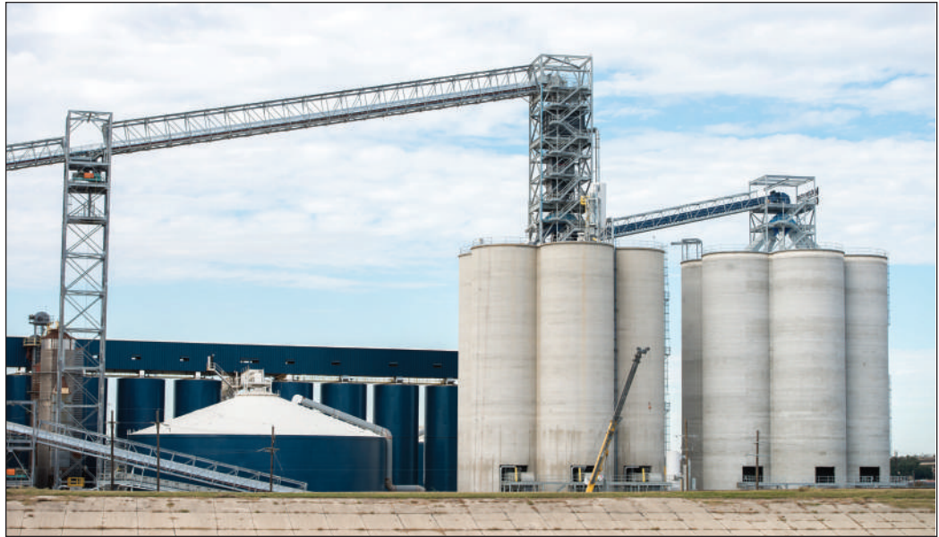
New shipping bins and bulkweigher nearing completing in January 2014 at the Louis Dreyfus Commodities export terminal in Port Allen, LA. Photo courtesy of T.E. Ibberson Company.
