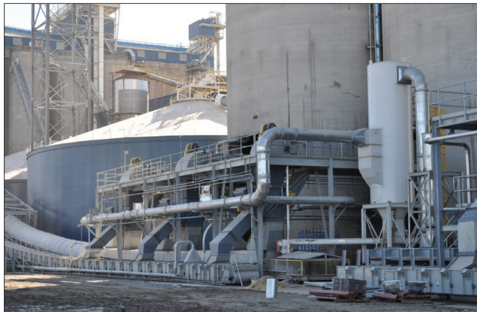
Unloading systems carry grain via gravity from seven hopper-bottom shipping bins onto an Intersystems enclosed belt conveyor running out to the dock. Photo by Ed Zdrojewski.
