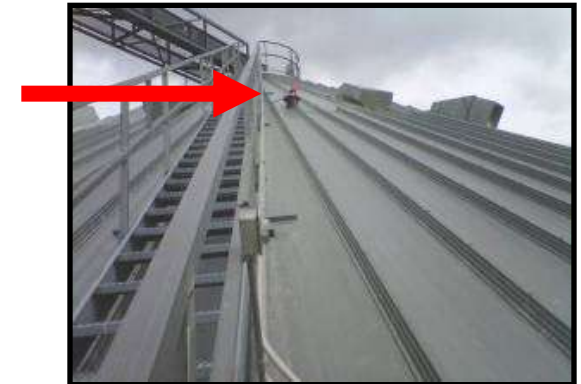
Scanner #2 mounted halfway between the center and sidewall.
