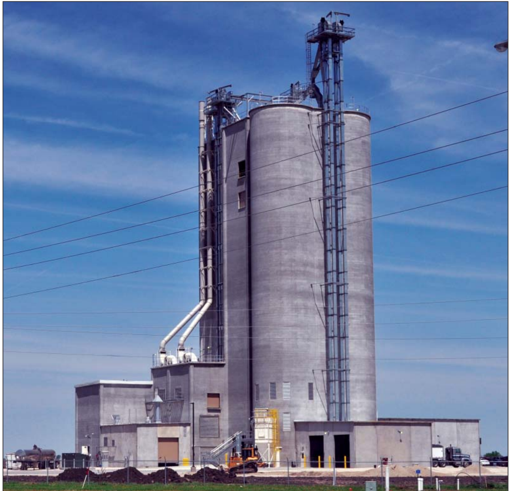
Cargill Pork's new $29 million 350,000-tpy swine feed mill at Hedrick, IA, part of a $60 million pork production investment Cargill is making in southeastern Iowa. Photos by Ed Zdrojewski.
