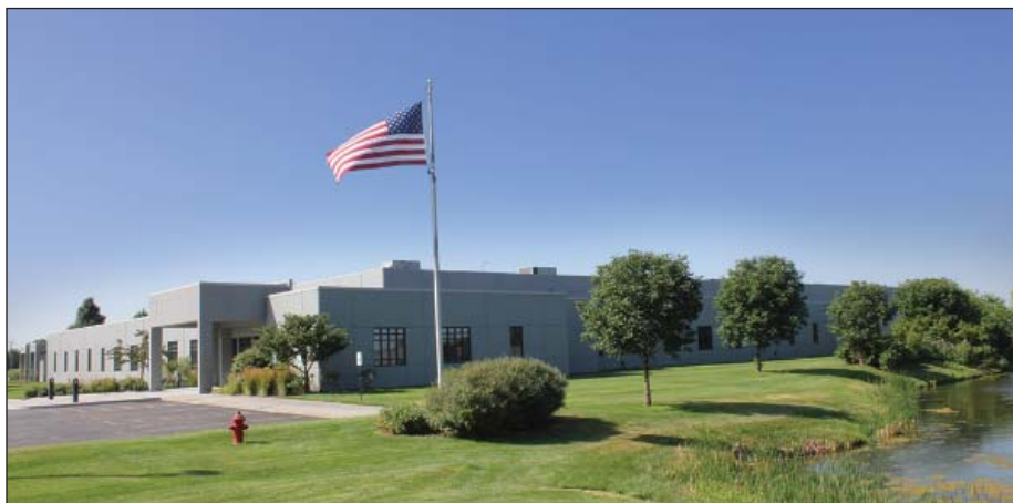
BinMaster's 75,000-sq.-ft. office and manufacturing facility just outside Lincoln, NE.
