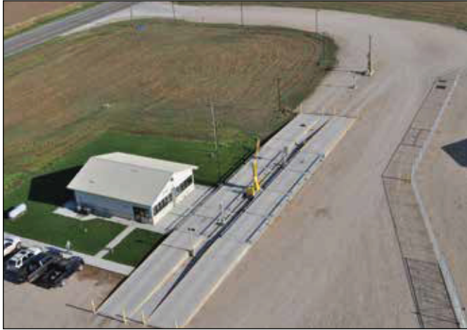
View from the elevator roof of the facility office and grain grading lab, with inbound and outbound Mettler Toledo truck scales and a pair of Gamet Apollo truck probes.
