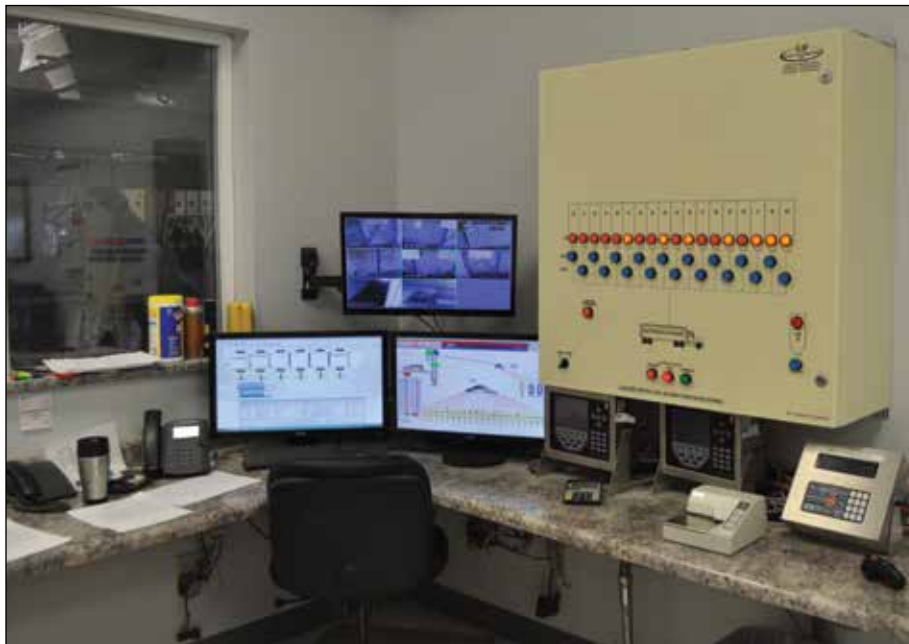
Control room features an Easy Automation batching system, which also is used to run a new grain elevator next door.
