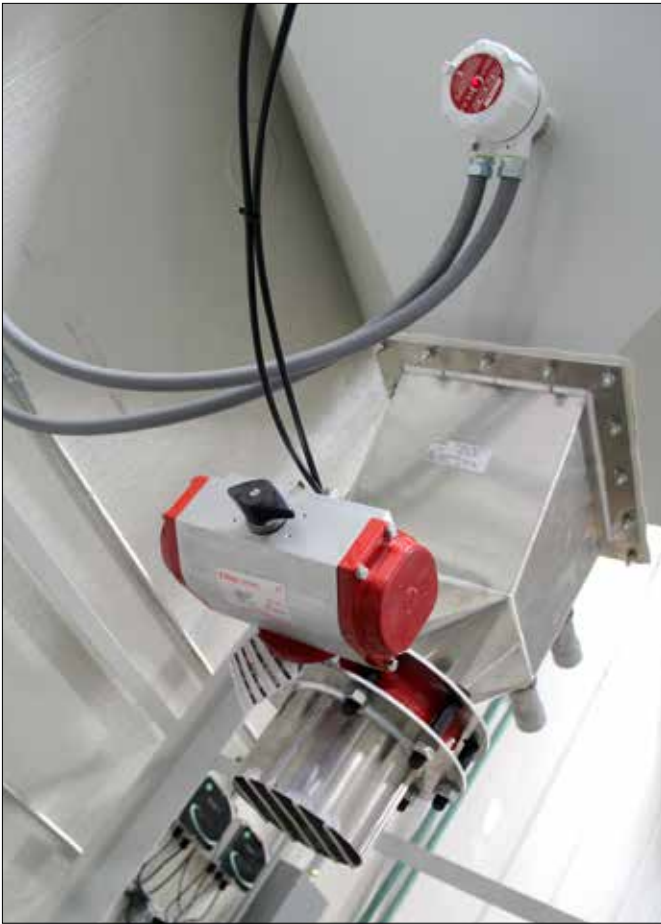
A standard vibrating rod is used in the cone of the surge bins to alert when resin levels are low.
