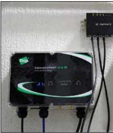
Wireless gateways eliminate long spans of wiring through the plant.
