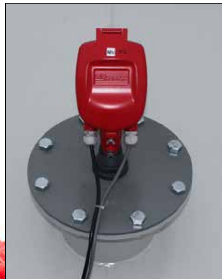
A 3DLevel-Scanner non-contact sensor mounted on the silo roof continuously measures the level of resins in the silo.
