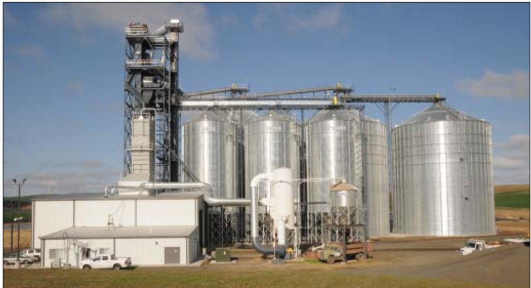
New McCoy Grain Terminal LLC rail terminal along a state-owned short-line railroad at McCoy, WA features 1.3 million bushels of upright steel storage. Photos by Bruce Selyem.
